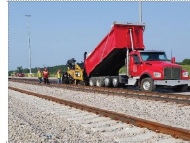
Lane paving between tracks 2 and 3
