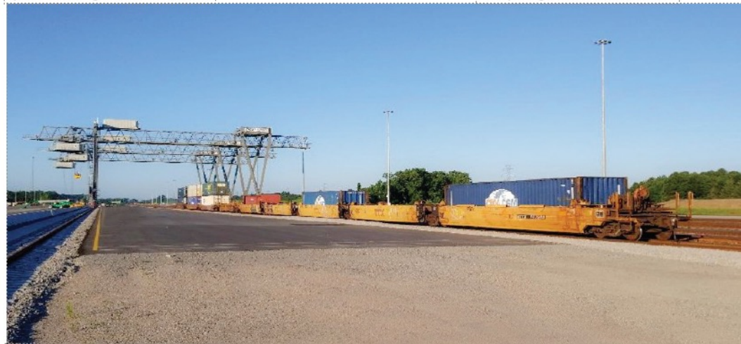
Cars and containers on site for crane testing
